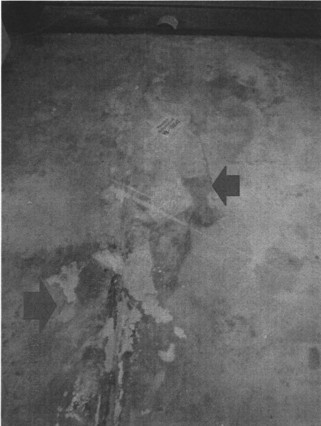
Millboard backing found on the concrete substrate floor within the Sch. 30 Kindergarten
