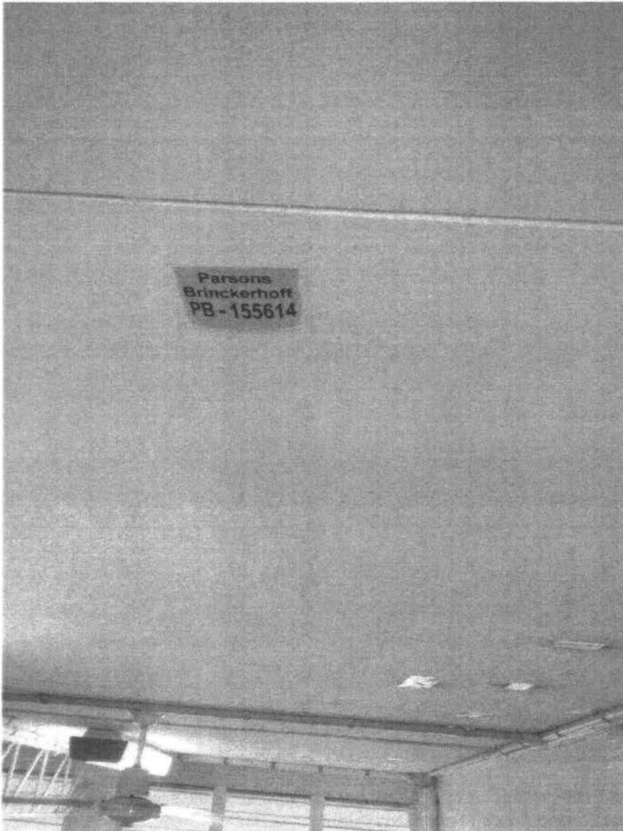
Sample PB-155614 Low density board ceiling in Room B6
