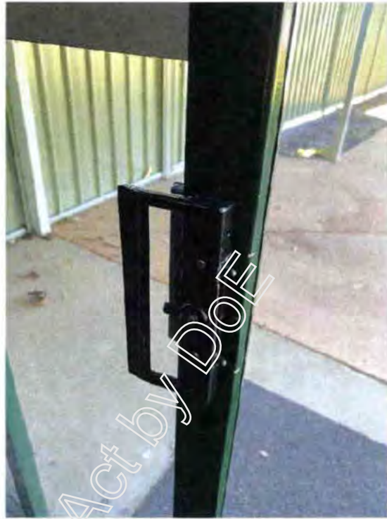
Non-compliant door hardware for PWD access
