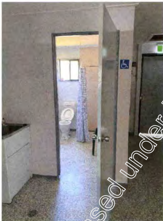
Access to PWD sanitary facility is non-compliant
