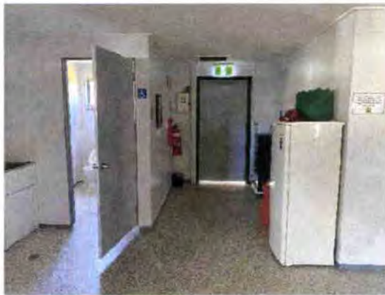
Internal public corridor to rear exit door is required to be fire rated
