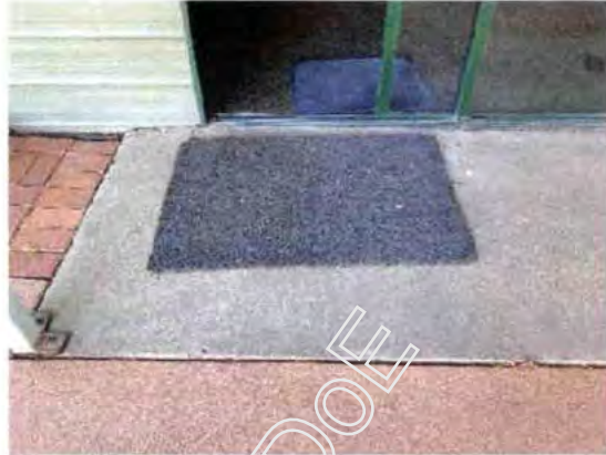
Door threshold at main entry should not incorporate a step
