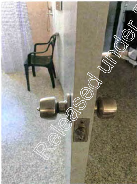
Door hardware needs to be upgraded to meet compliance with current standards
